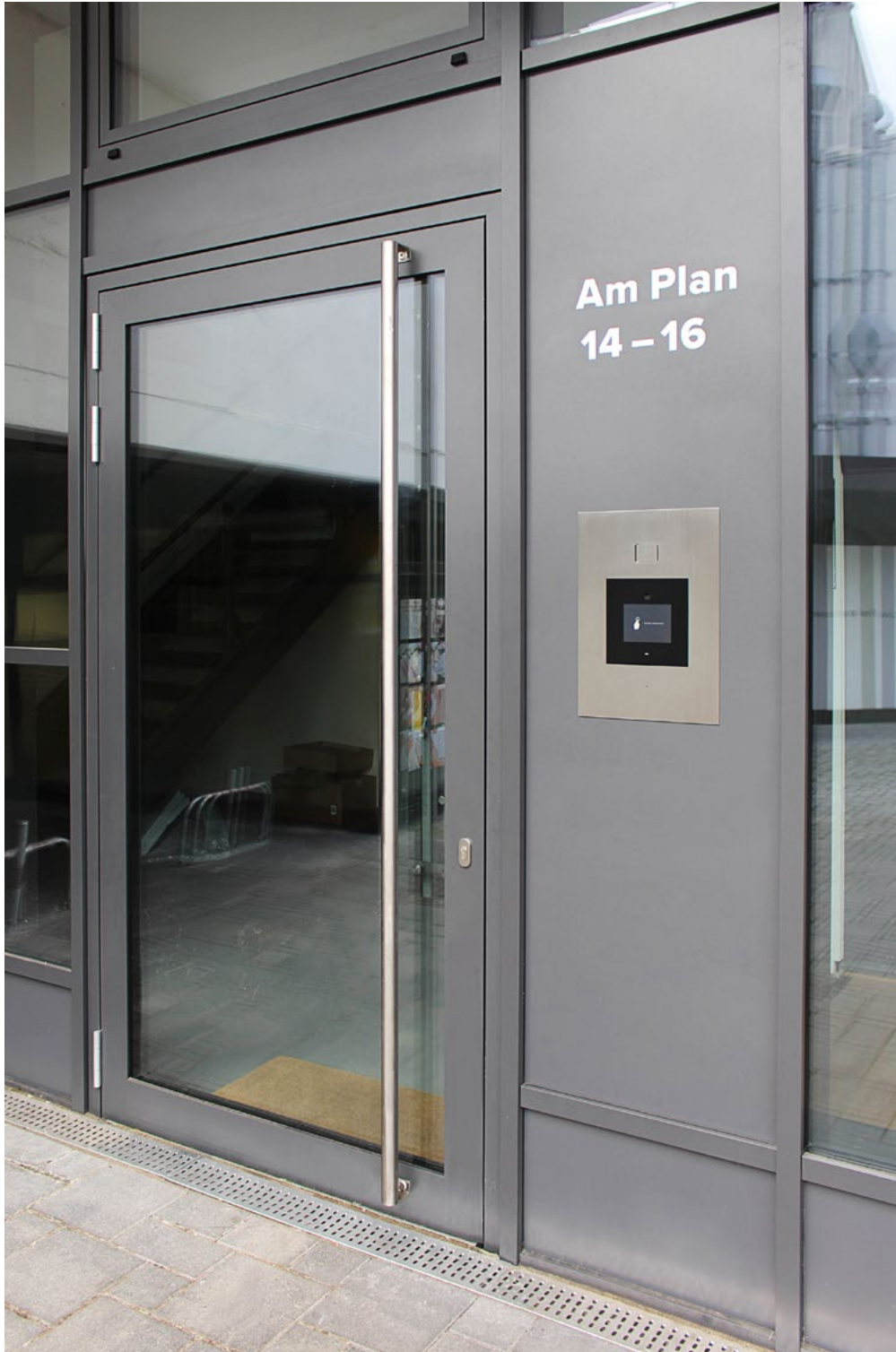
Front panel stainless steel brushed, installation in a door side panel
